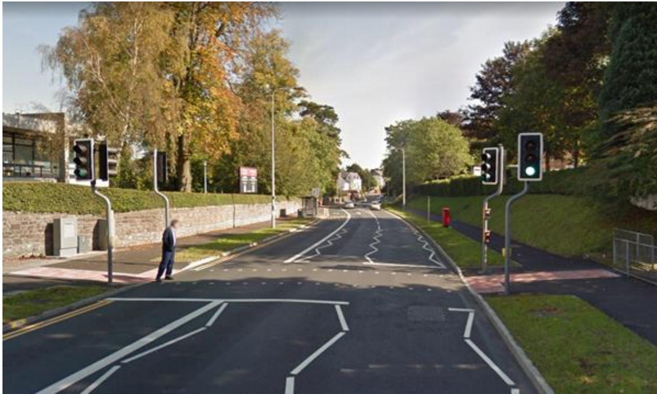
Llantrisant Road, between Bridge Road junction and Danescourt Station
