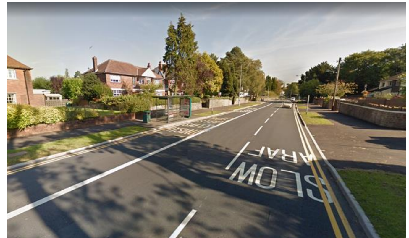
Llantrisant Road, between Bridge Road junction and Danescourt Station
