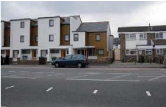
This contemporary redevelopment of a former garage site comprises of three-storey terraced housing.
