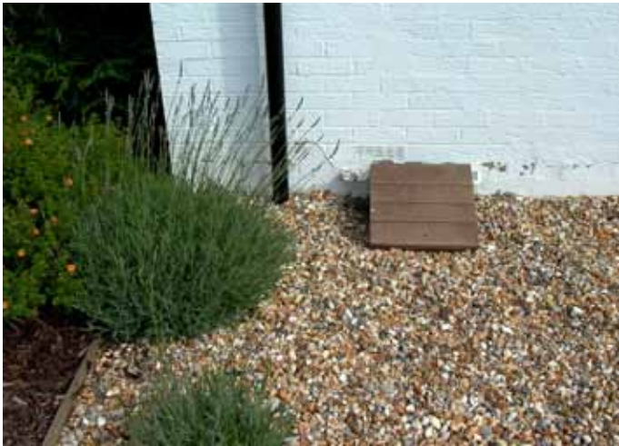
44. Locate utility meters in the public realm, but not as a prominent feature on a building facade
