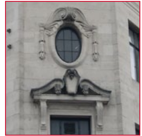
Carved stone around openings, 2 Queen St.
