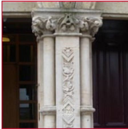
Carved Bathstone pillars support arched doorways.
