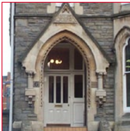
Decorative pointed arch, and Bath stone hood over recessed doorway – Park Place.
