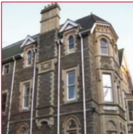
Park Place – the corbelled chimney stack and windows add interest to the side elevation.
