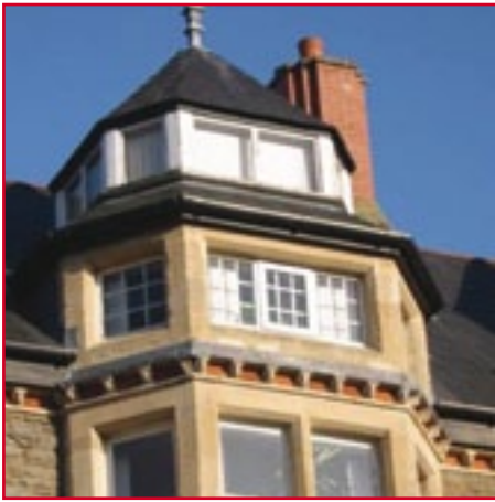
The bay windows of 3 – 4 Park Place are topped at attic level by a pyramidal roof.
