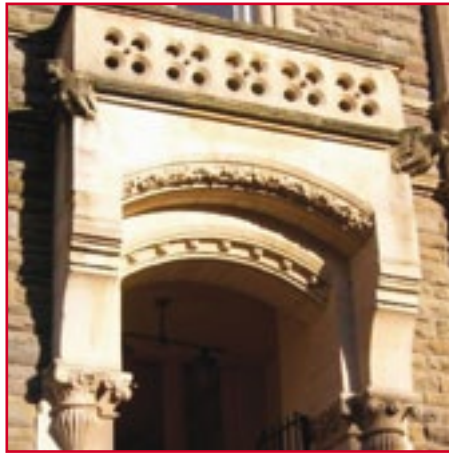
Bath Stone hood over doorway with ornate detailing including a fretted parapet and figurative carvings.
