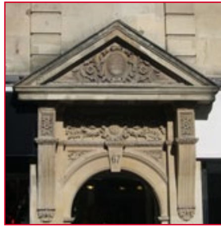
Carved stone over door-way, the Andrews Buildings.
