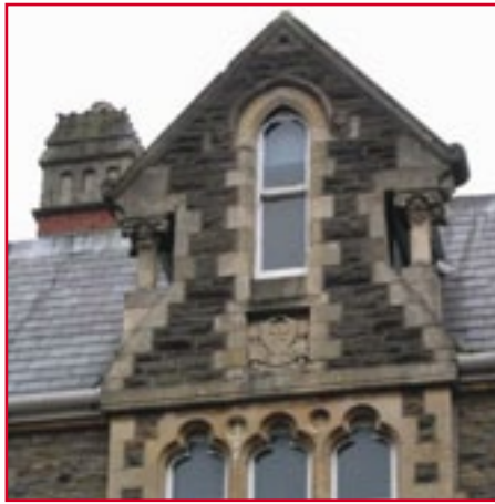
Dormer and chimney detail at 5 & 6 Park Place.
