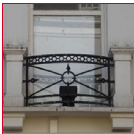
Convex iron frontal across first floor window.
