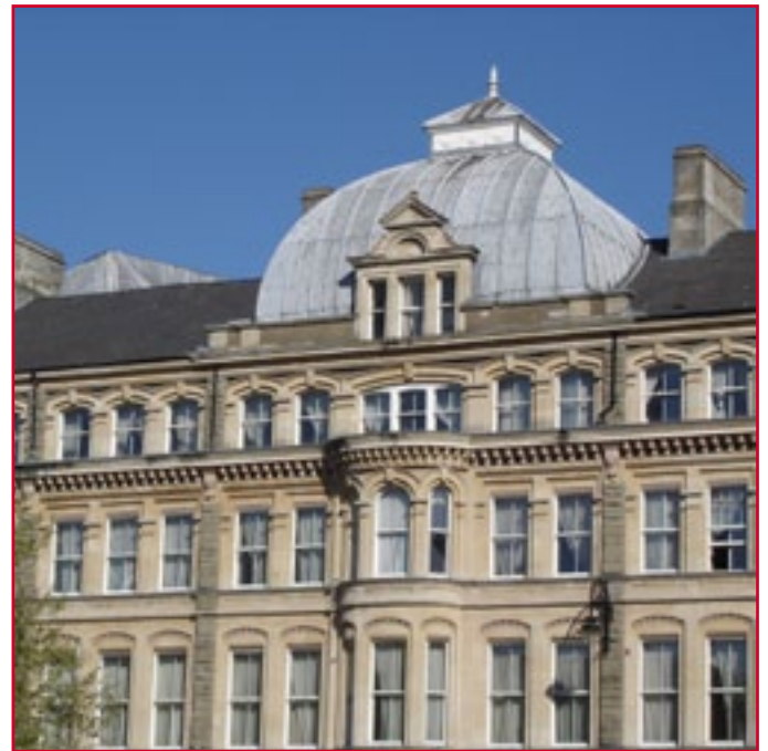
Park Hotel, Park Place / Queen St
