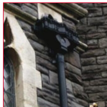
Cast iron rainwater head and down pipe – City United Reformed Church.
