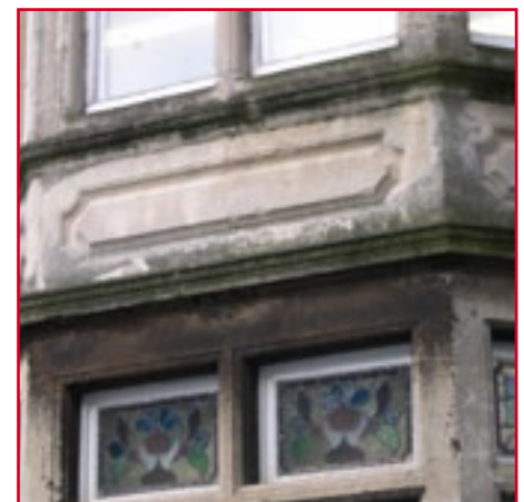
Leaded lights within a stone bay.
