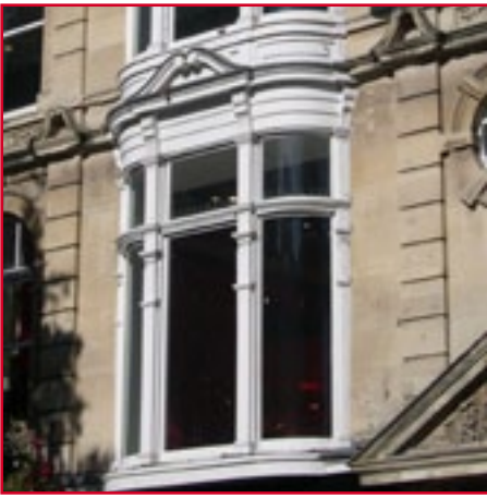
Victorian window detailing at the Andrews Building.
