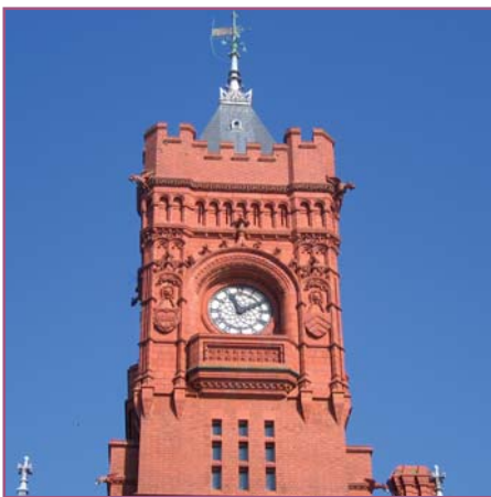
Clock tower featuring parapets and gargoyle architectural detailing, Pierhead Building
