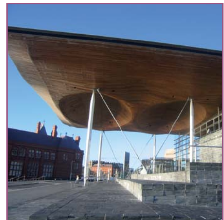
Timber detailing on the underside of the roof of the Senedd
