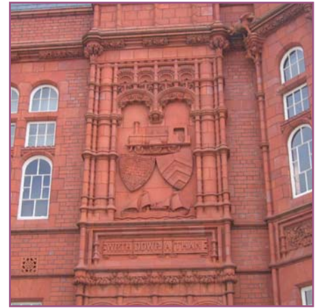
Red brick walling displaying detailing combining both the Medieval Gothic and French Renaissance styles, Pierhead Building
