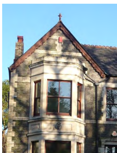
Decorative bargeboard and grey slate roof, Cardiff Road.
