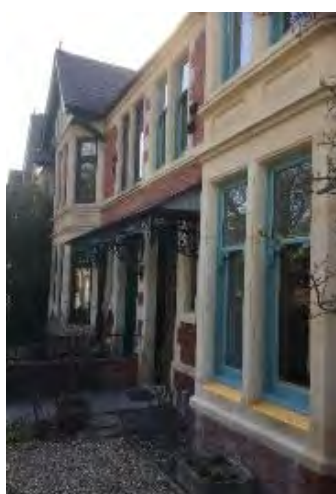
Cast iron and glass porches, Cardiff Road.
