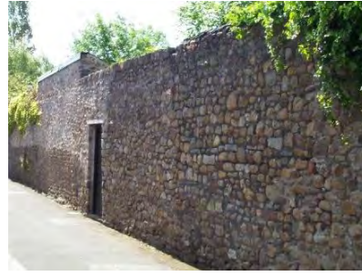
Historic rubble stone wall.
