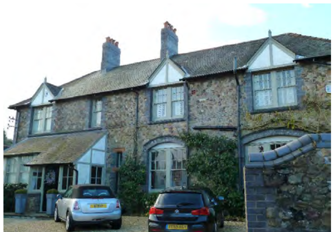
Polychromatic random rubble, pennant band courses, Staffordshire blue brick voussoirs and quoins: Heol-y-Pavin.
