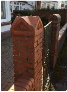
Brick pillars, decorative coping.
