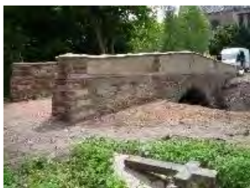
Prichard Bridge repair and refurbishment in 2012/13.
