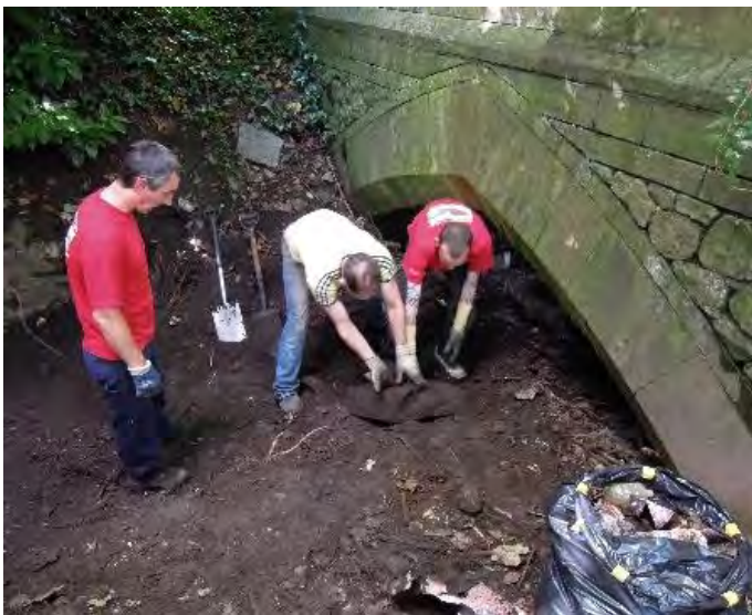
Prichard Bridge (2013) Restoration project.
