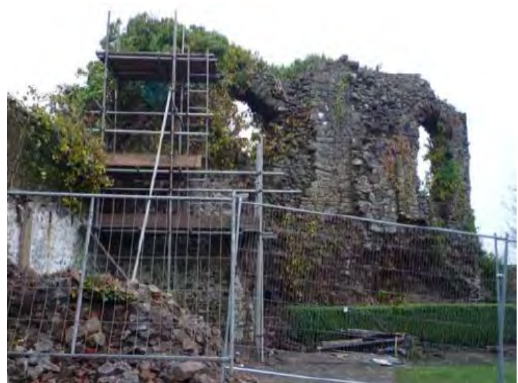
Bishop's Palace (2012) survey work, vegetation removal, repairs and interpretation
