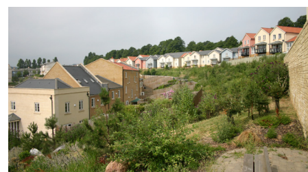
A variety of buildings and roof-types create enclosure, an interesting sky-line and respond to site-specific topography and landscape context in Portishead.
