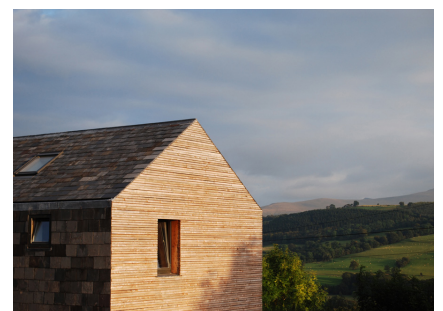
Sustainable building sensitive to context, Ty Pren, Powys, www.feildenfowles.co.uk/projects/typren
