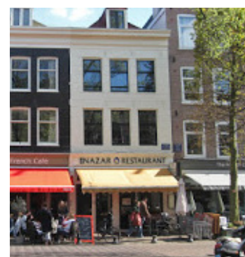
Flats above shops, 3-5 storey Amsterdam.
