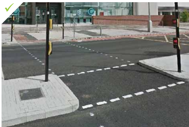
Straight across crossing at Adam Street
