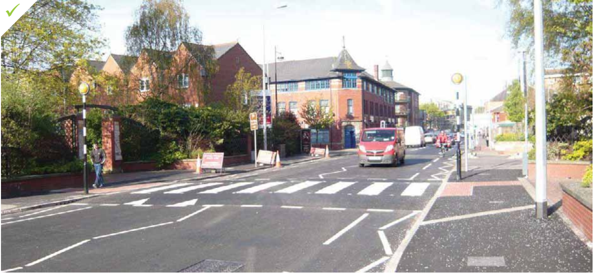
Raised table macadam crossing at James Street
