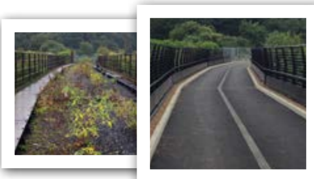
Cart Road 52 – Before and after
