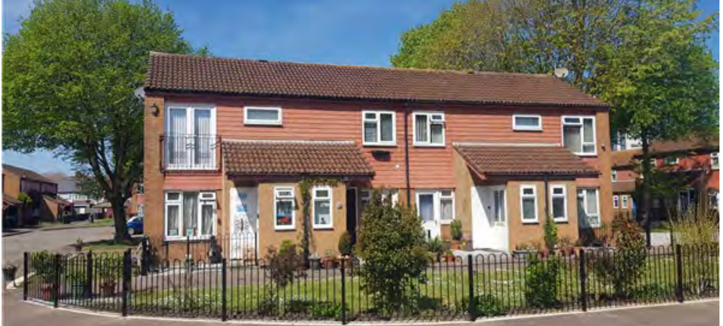
Regeneration works to Taff embankment
