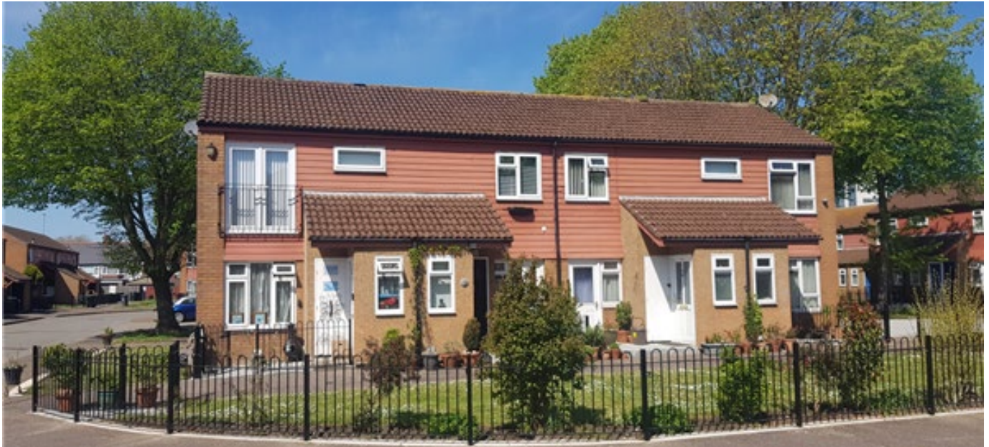
Regeneration works to Taff embankment
