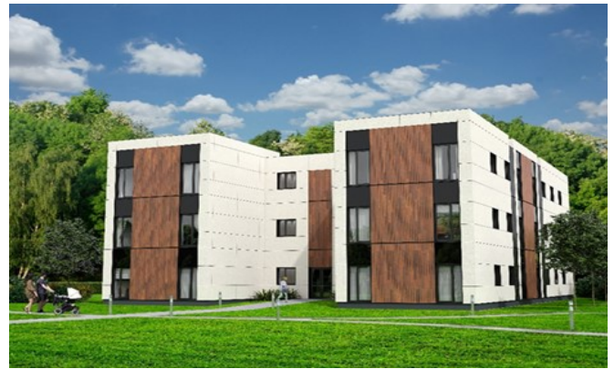
Gas Works site, Grangetown - new supported accommodation for families.
