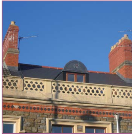
Dormer atig crwn, simneiau brics coch a manylion Carreg Caerfaddon, Windsor Esplanade
