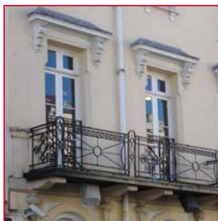
Balconi haearn gyr ar draws tri drws ffenestr o gan gornisau braced.
