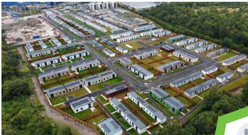
Gasworks modular builds site
