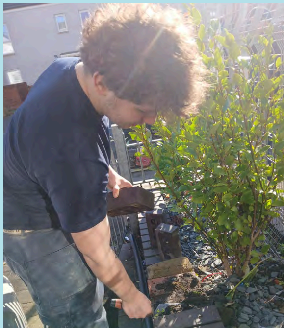
Repairs Academy apprentice Jason at work
