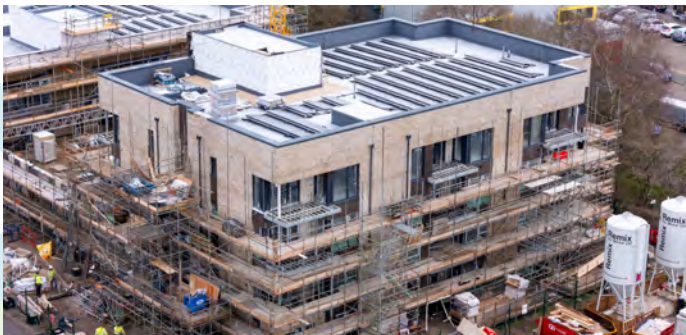
Construction of St Mellons Community Living
