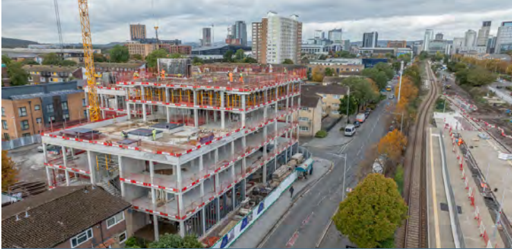
Construction of Bute Street Community Living
