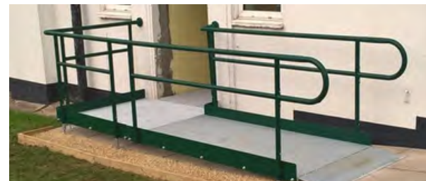
A ramp allowing for access to a wheelchair user
