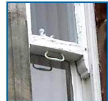
Most of the benefit which accrues from fitting new windows, is that they are less draughty than older windows. Sometimes the fitting of a modern draught stripping system is less costly and will be as efficient as the insertion of new windows. They are known as weather strips or brushes and can also enhance noise insulation, ease rattling and the operation of windows. In some cases secondary glazing in a removable inner frame is another alternative.
