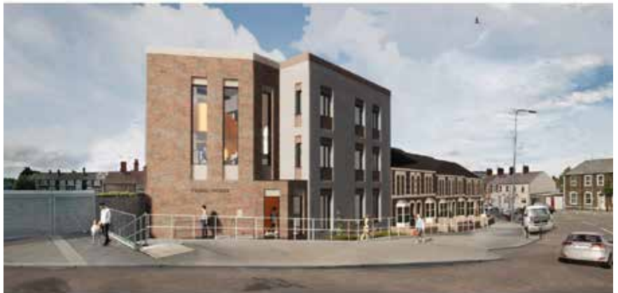
Pearl House, Splott Road Austin Smith Lord Architects
