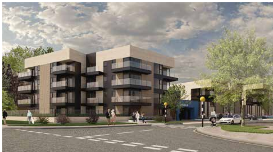
Former St Mellons Community and Education Centre C2J Architects
