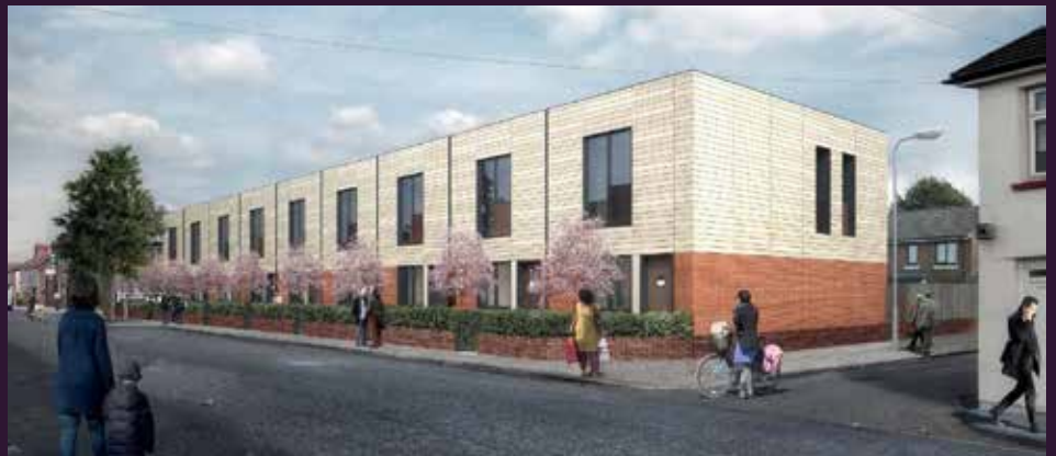
Crofft Street Housing Rogers Stirk Harbour and Partners
